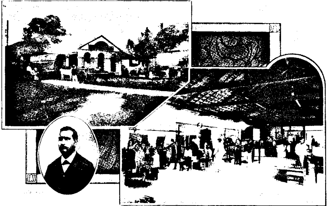
PURE ICE AND AERATED WATER MANUFACTORY—J. W. FERNANDO, AND VIEWS (INTERIOR AND EXTERIOR) OF THE FACTORY.
