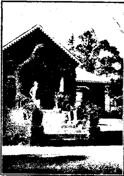
SUPERINTENDENT'S BUNGALOW, HORNSEY ESTATE, DIKOYA.
