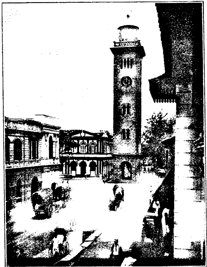
THE LIGHTHOUSE AND CLOCK TOWER, CHATHAM STREET.
