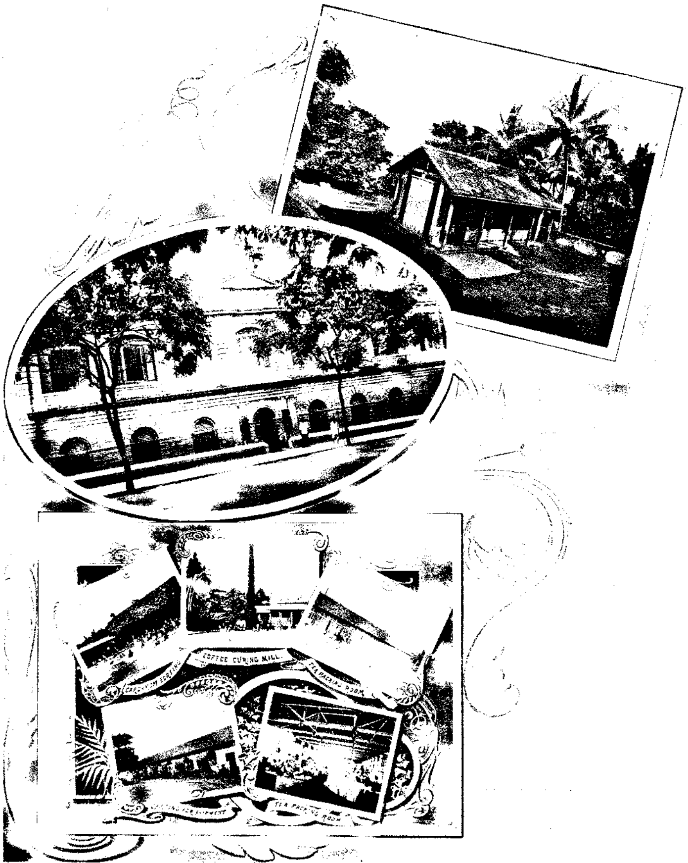
MESSRS. BOSANQUET & CO'S GENERAL OFFICE, DYNAMITE MAGAZINE, AND GENERAL VIEWS.
