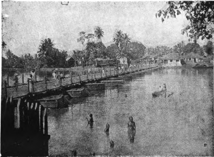
The Old Bridge of Bouts, Grandpass.
